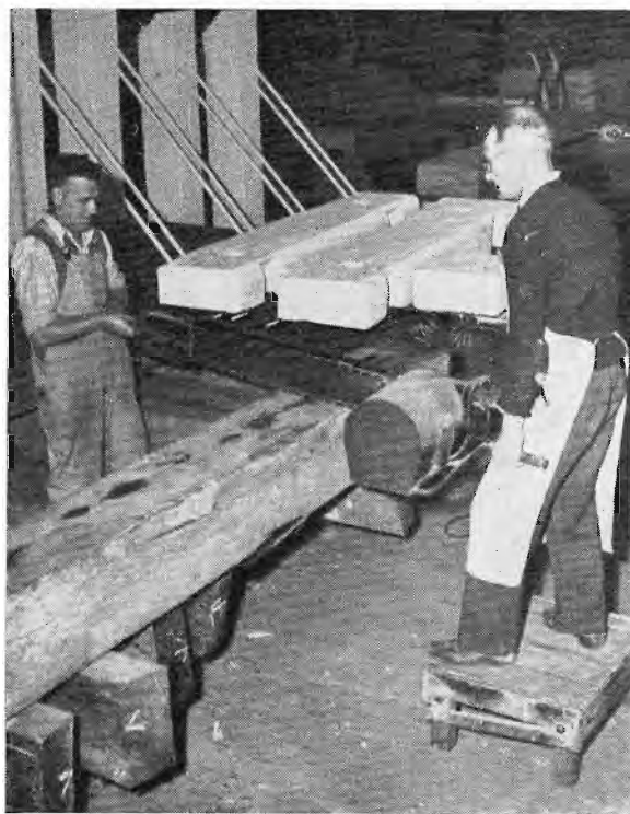
Buffer Stops being turned out.
