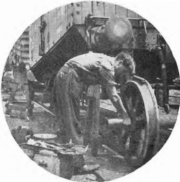
Typical activity in the lifting yard.
