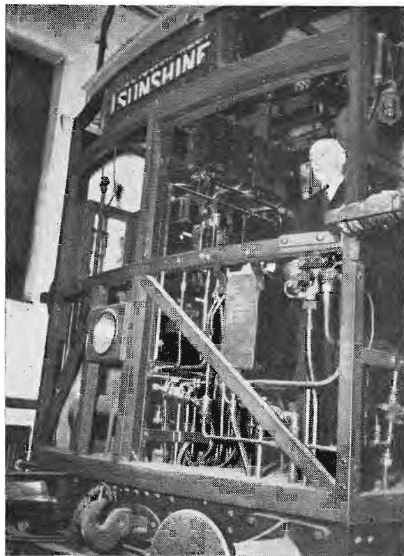
The skeleton coach used to teach Drivers at the Electric Running Depot.
