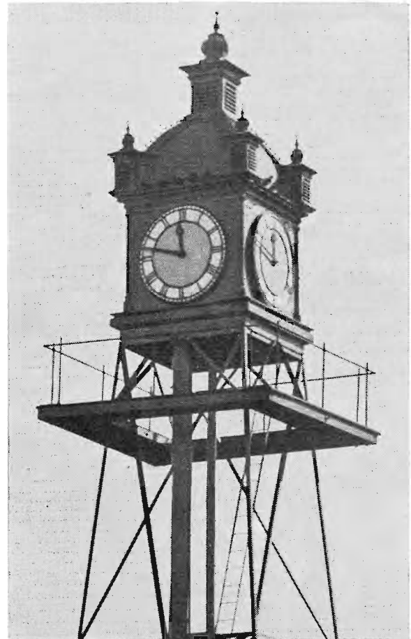
Spencer Street tower clock.
